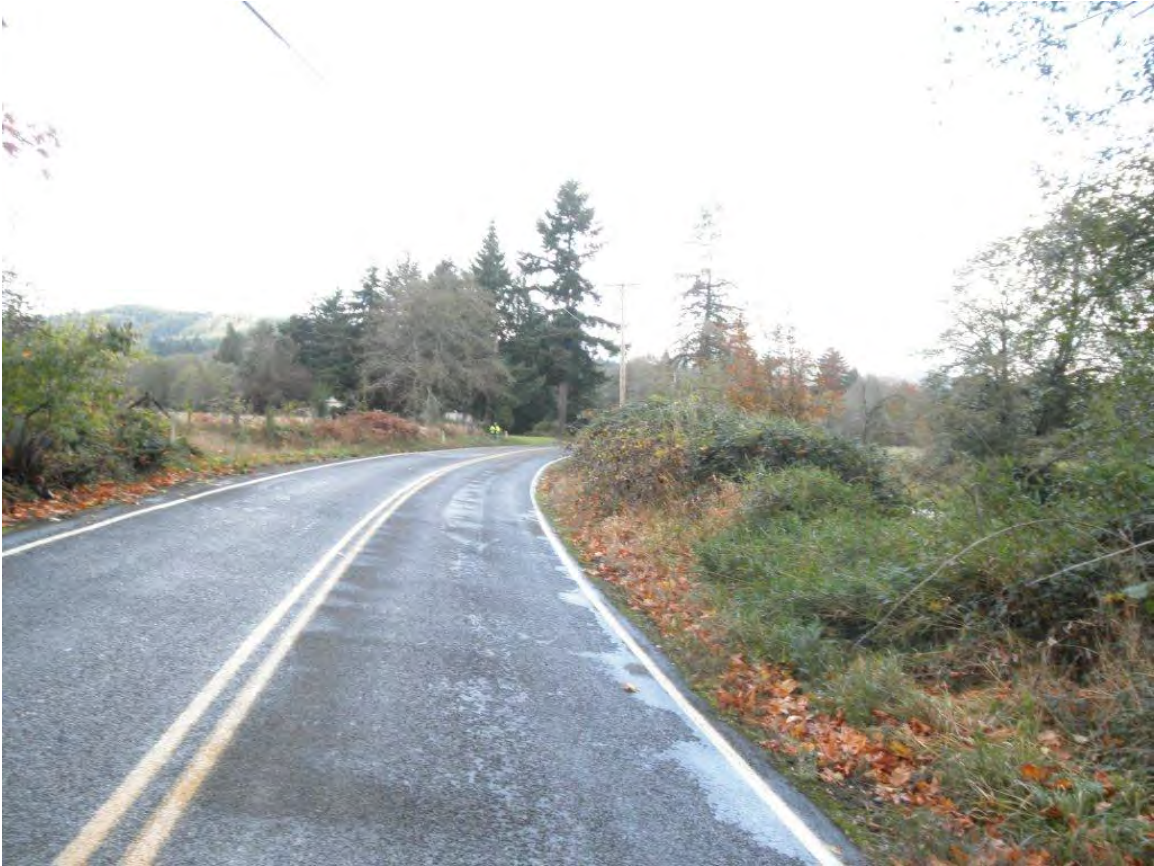
Limited sight distance at approximate milepost 5.03 Elochoman Valley Road
